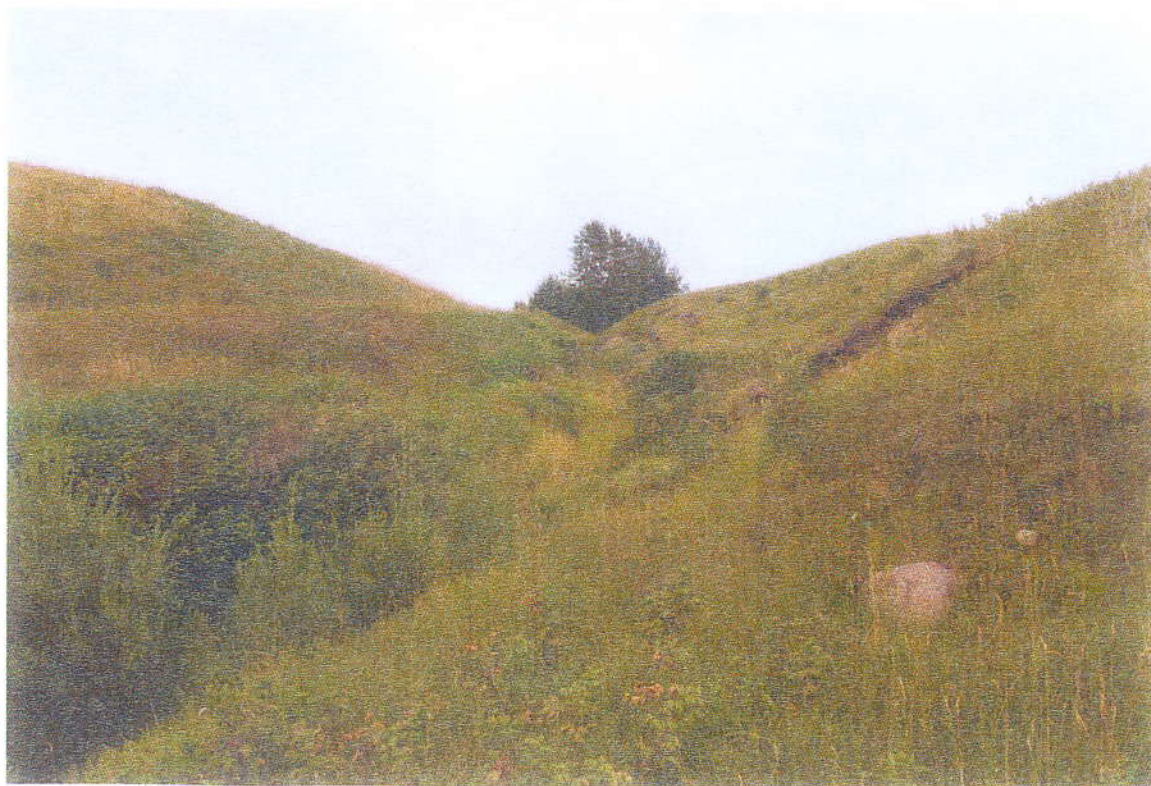
Water course that was eroding, now has willow, and spruce to support the banks. ( Small spruce are at the top, the willows are visible thru out)
