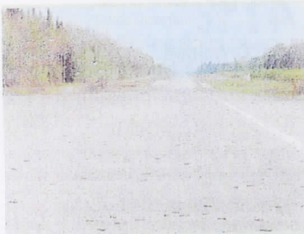
FTC on NW Alberta highway in 2005. Photo Mike Maximchuk
