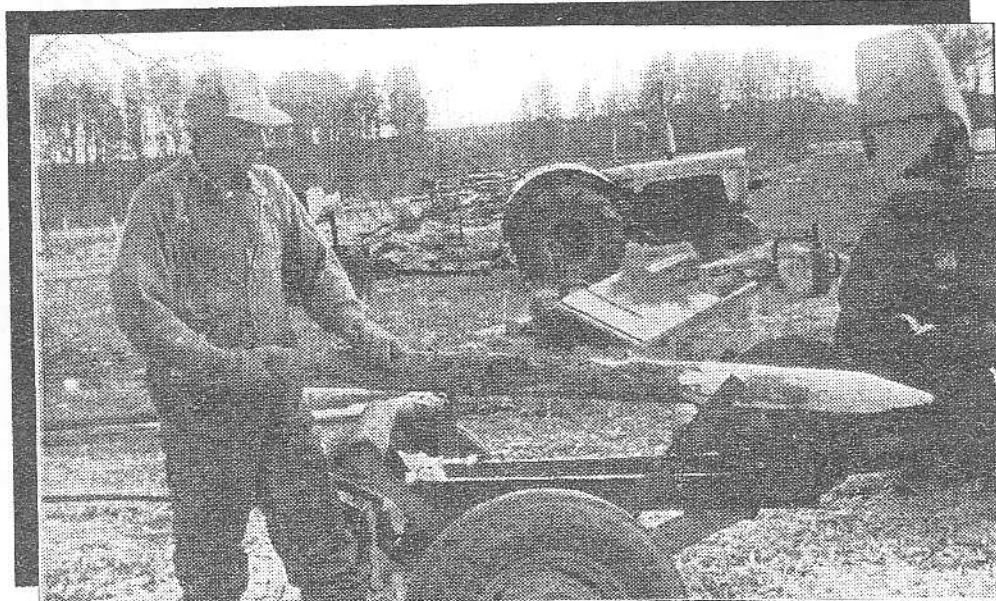
The Reddi-Post efficiently sharpens posts up to eight inches in diameter and will dedebark anything from two-inch fence posts to ten-inch corral posts.
