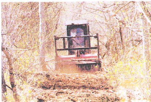
Figure 6 - Mulcher cutting new trail through native bush
